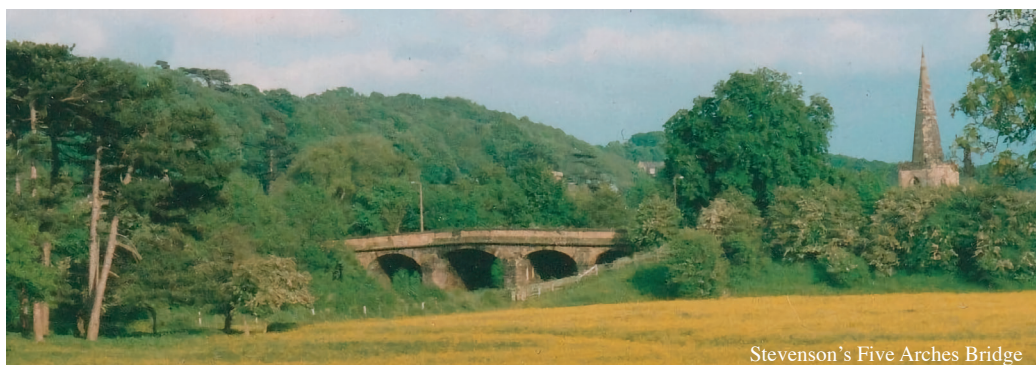
Stevenson's Five Arches Bridge
