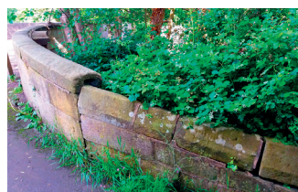
Duffield Bridge, old (right) and new coping stones
