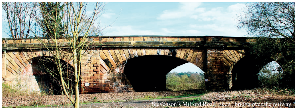
Stevenson's Milford Road 'skew' bridge over the railway
