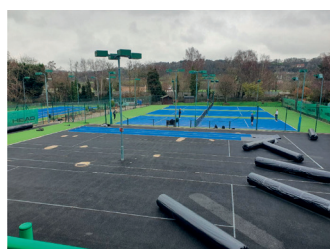
The second phase of court re-carpeting gets underway
