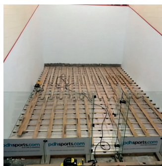
Work on the squash show court which now includes underfloor heating.
