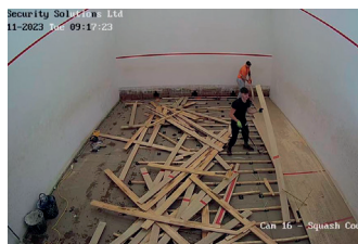
Ruined flooring being dismantled on one of the squash courts
