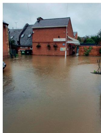
The car park under water
